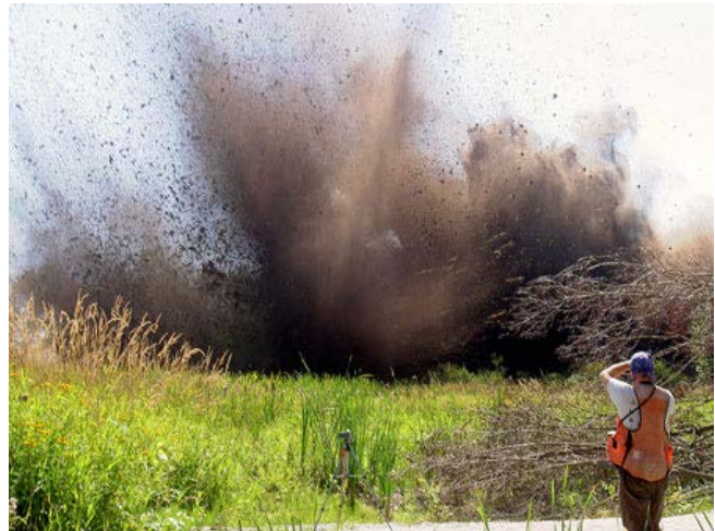
Excavation of interior marsh channels using explosives. Photo credit: Skagit River System Cooperative.
