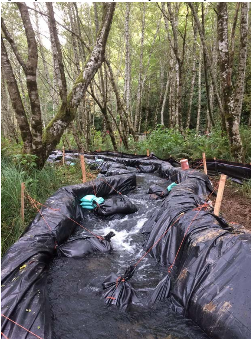
Temporary channel during construction.
